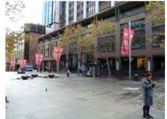
EXISTING view - looking northwest toward 60 Martin Place
