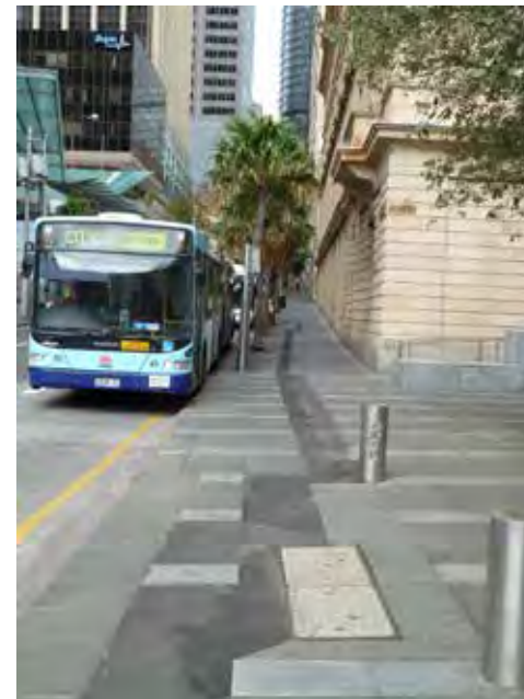
Young Street view south - existing
