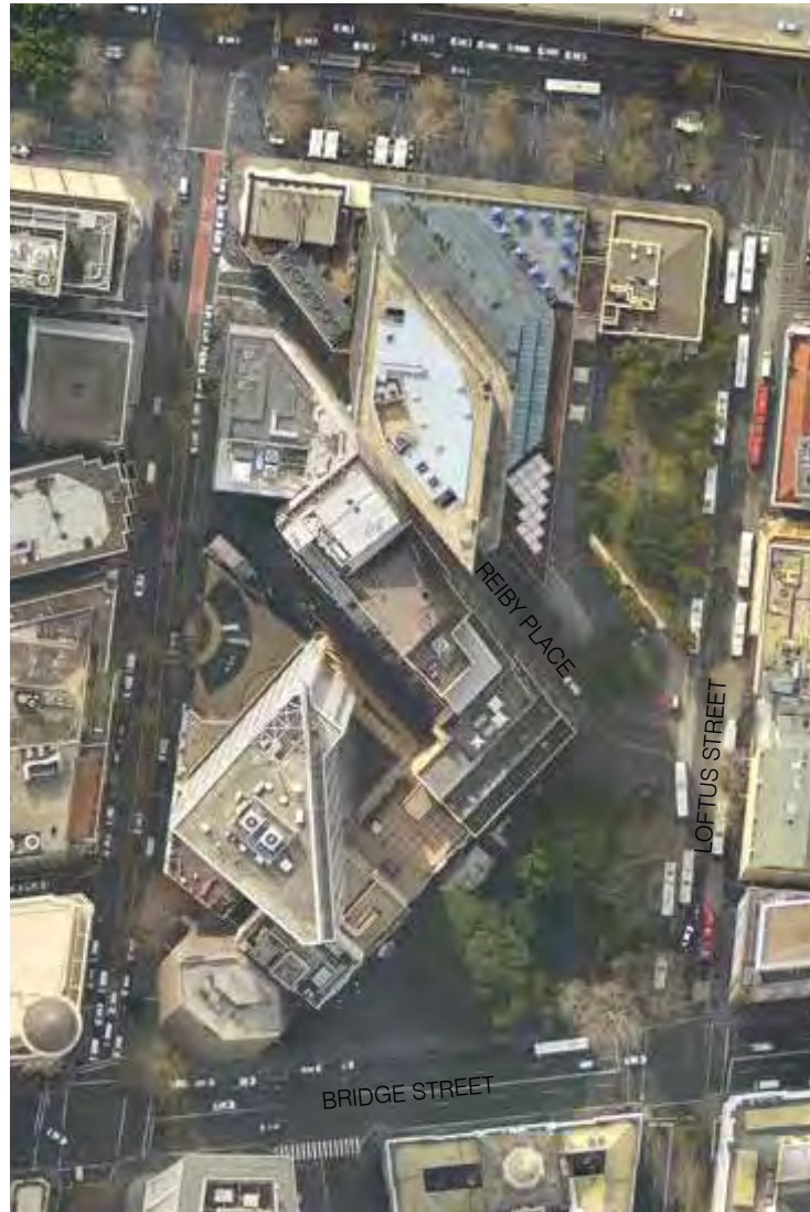
Loftus Street and Reiby Place - existing
